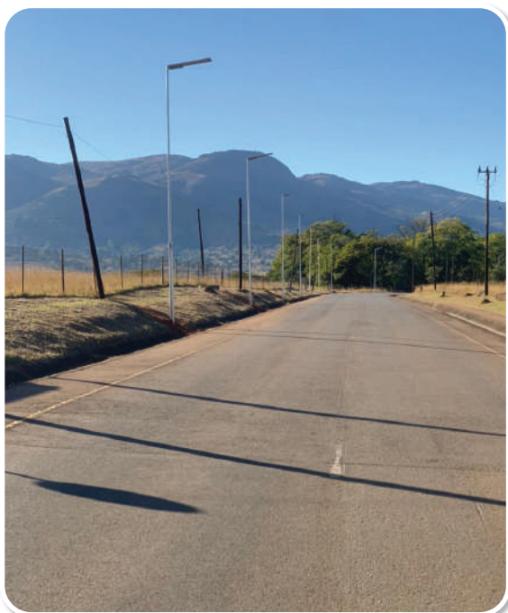
Figure 1: Installed solar-powered streetlights at Mantenga Drive and Mpumalanga Road, Ezulwini.
