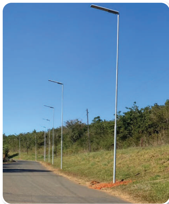
Figure 1: Installed solar-powered streetlights at Mantenga Drive and Mpumalanga Road, Ezulwini.
