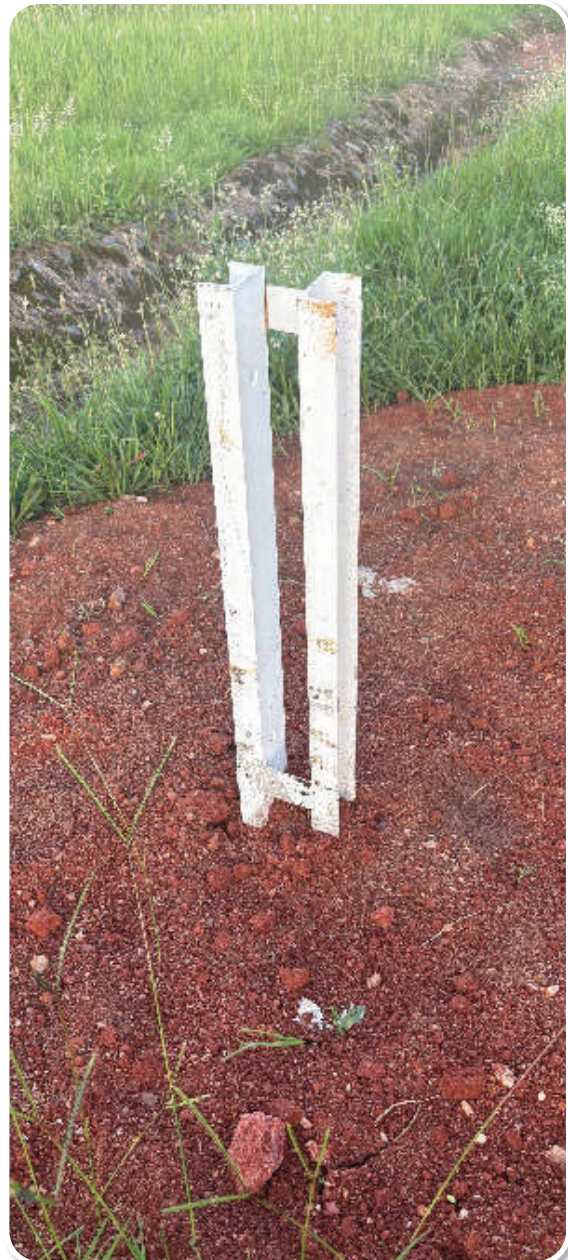
Image 7: Installed flag pole channels
